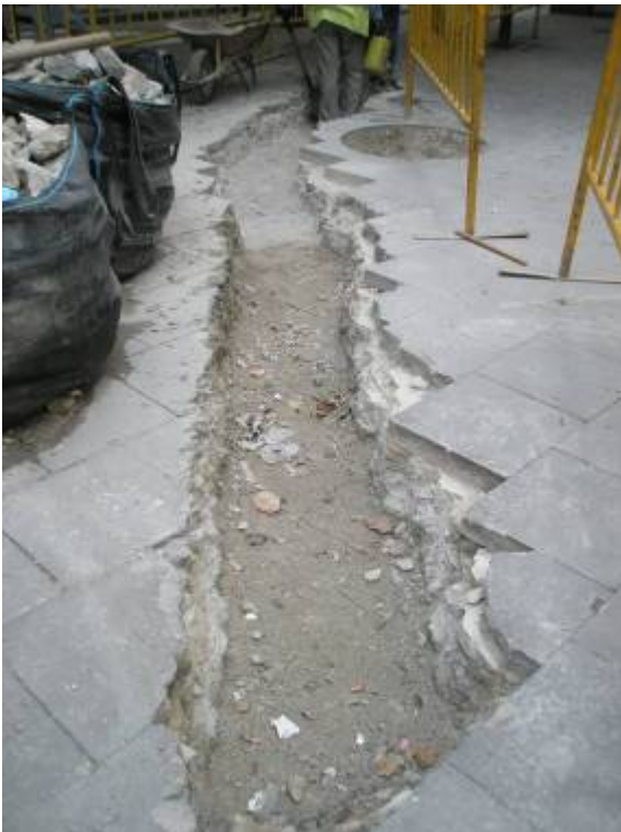
Obertura Tram 1, Rasa 100
